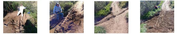
The February Trail Blazers trail work party was held on the Mt. McCoy trail. Work was conducted in 3 areas. The first area was at a steep sharp turn in the trail that had been rebuilt with rock on two previous work parties and both times were collapsed by hikers short cutting the turn. This time we installed an 8 foot section of 2 x 8 board. The board was backed up on both sides by rock and then covered with dirt. Brush was trimmed on the turn as well, to encourage hikers to stay on the trail.
